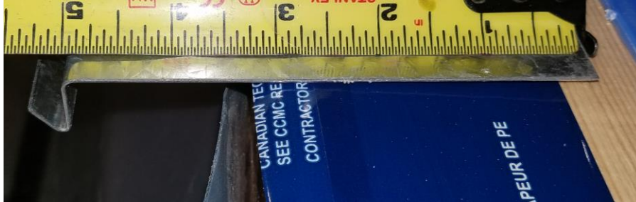
Head track profile, along the top of assembly
