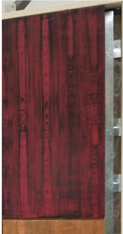
Continuous Z-track on right side of assembly
