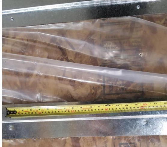
Screw spacing for horizontal tracks
