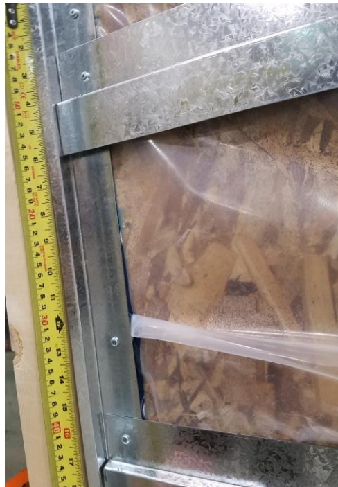
Screw spacing for left vertical track
